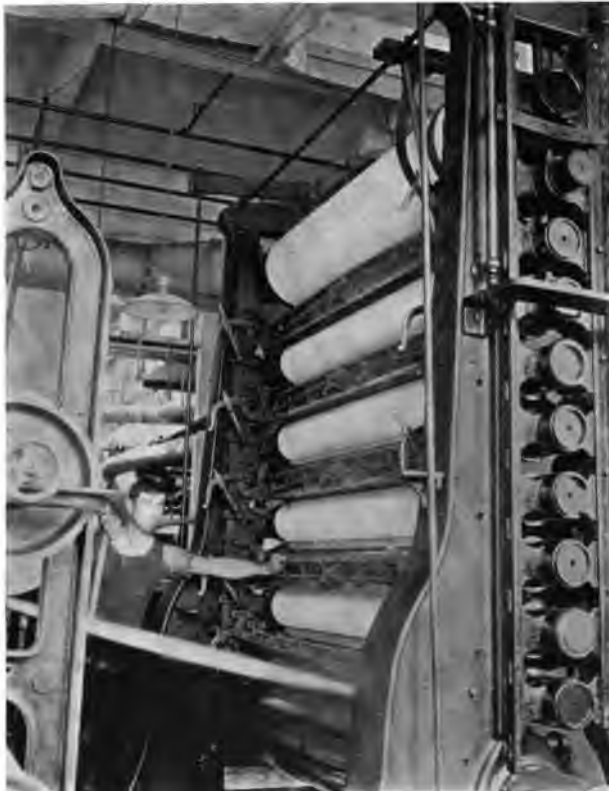
Fig. 2. Calender with Ribbon and Doctor Feed.
